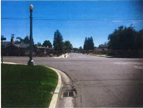
Photograph 1: Looking south from Merrit Avenue, Source 4-Creeks 4/3/2017
