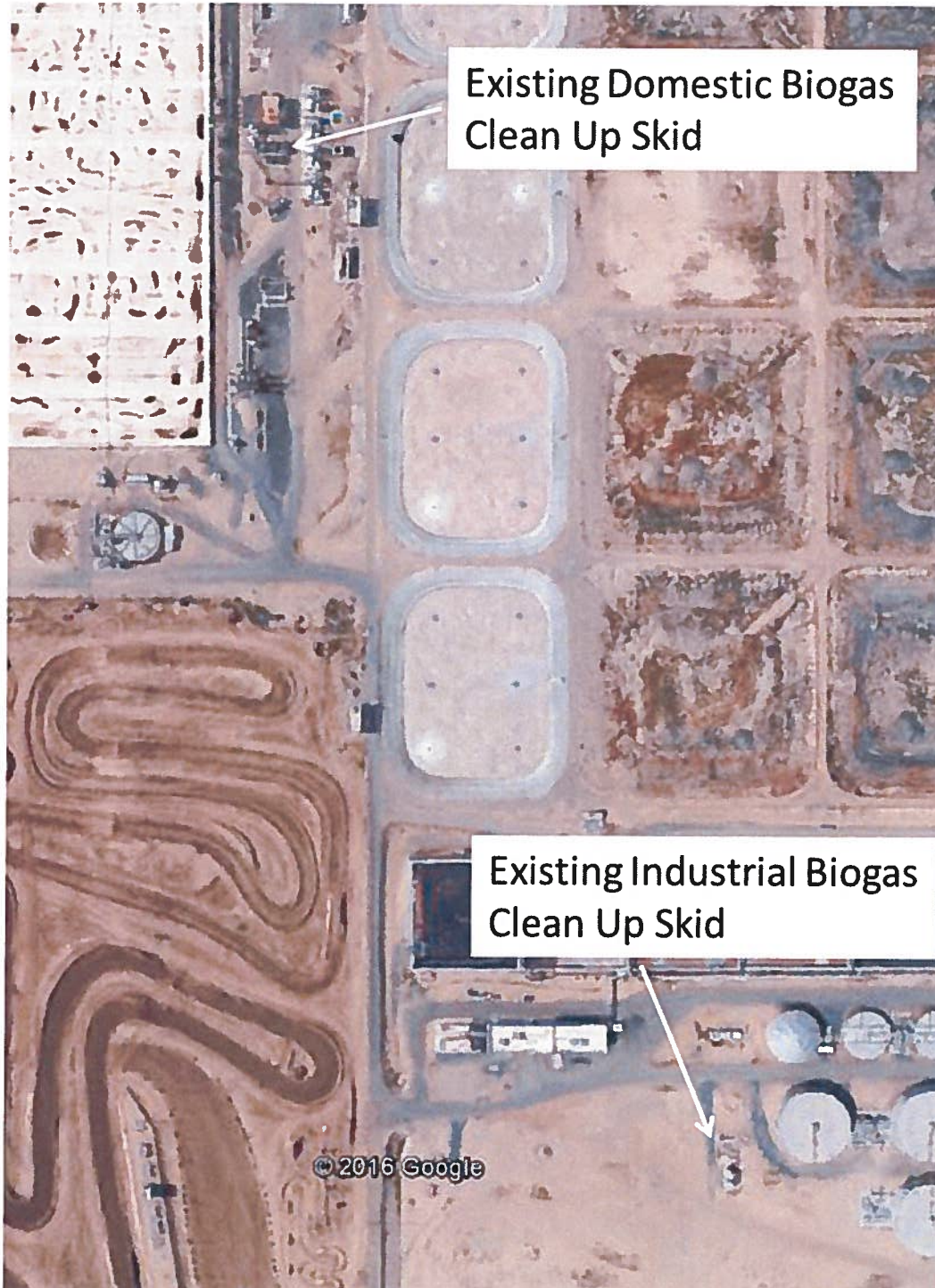
Figure E- 1 Locations of the Existing ADG Cleanup Equipment at Tulare WWTP
