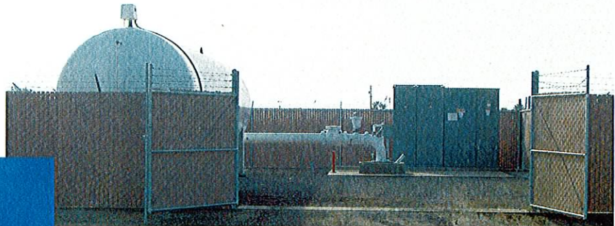
Right: Installation of Water Well Site 42
