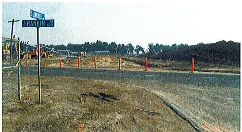
The construction of the new Dale Fry Road
