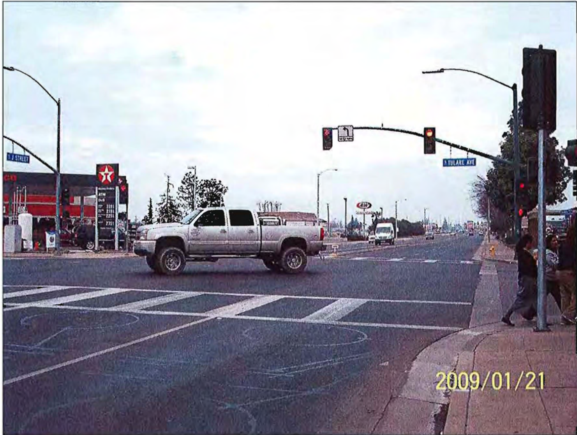
After several years in the planning, Engineering staff oversaw the reconstruction of J Street.
