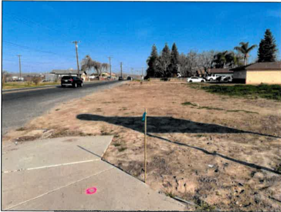
View of the take area looking north along the West Street frontage from the southwest corner of the parcel.
