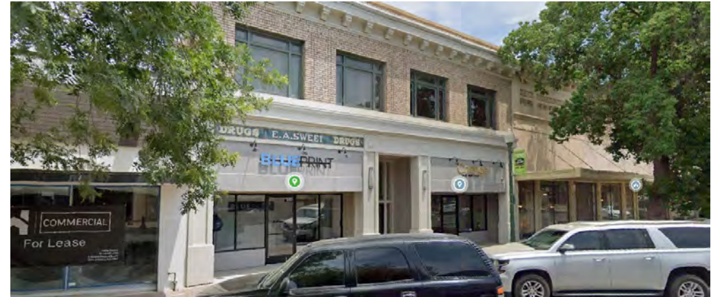
K Street Building Rehabilitation
