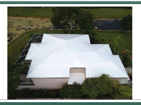
The 12-mil-thick polyethylene film is heated to shrink to the roof, securely wrapping it to create a fully-functioning, leak-free roof that can stay in place for up to 12 months, resisting water and wind and preventing further damage.
