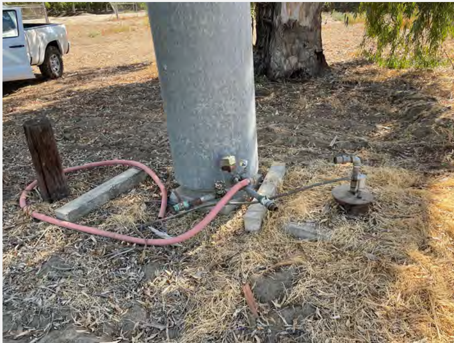
45. Abandoned domestic groundwater well located in vacant area along western subject property boundary.
