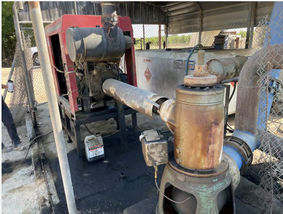
41. Diesel AST and motor located adjacent to one of the irrigation supply groundwater wells.
