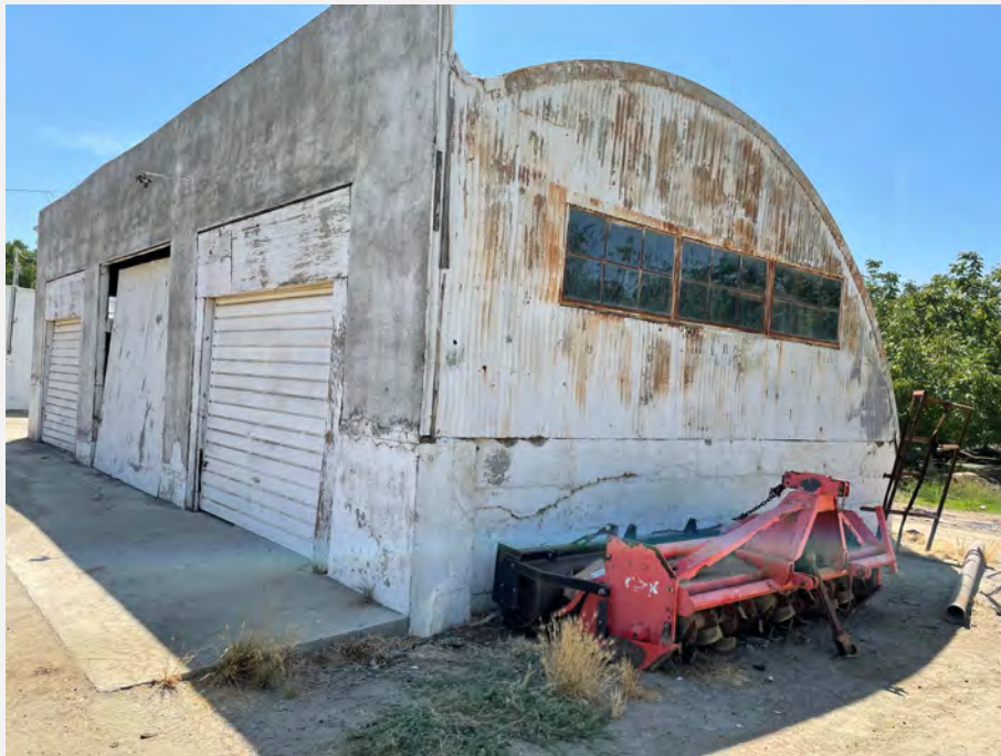
11. Outbuilding behind residential structures on the north-central subject property boundary.
