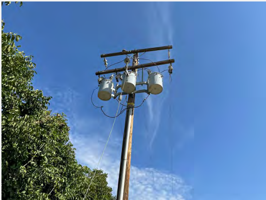
46. Pole-mounted transformers supplying power to electric pump at the irrigation supply groundwater wells.
