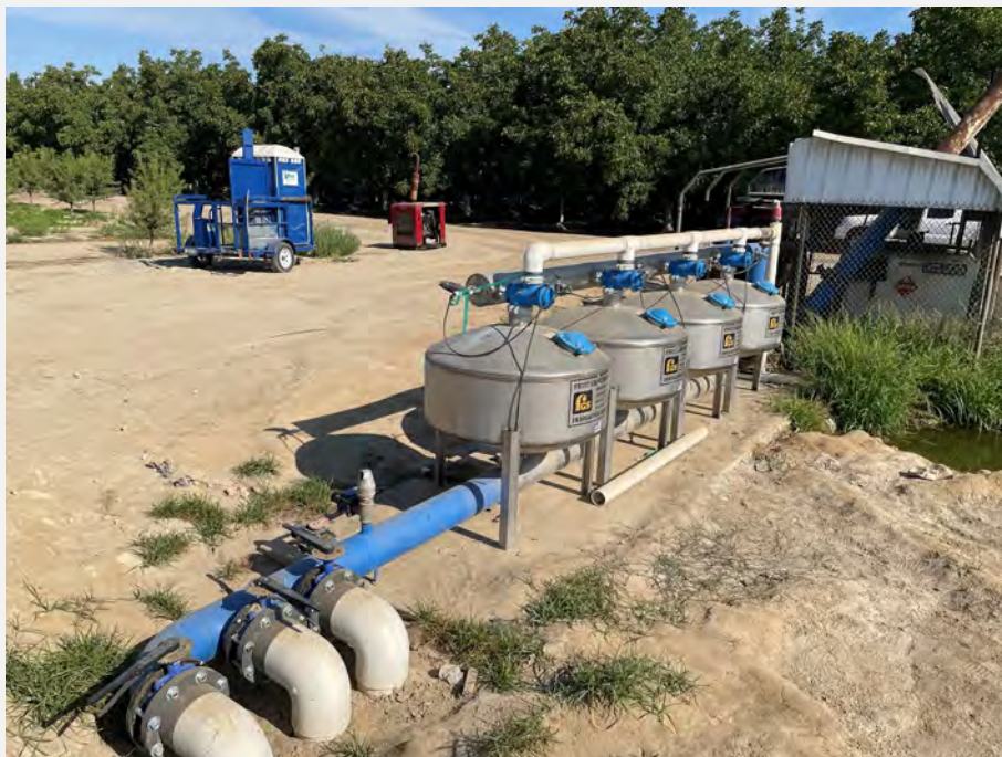
40. Filtration system located adjacent to groundwater wells.
