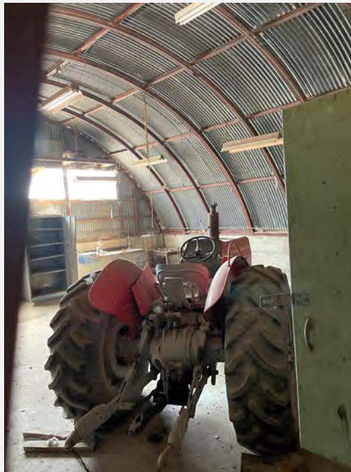
15. Interior of outbuilding. Access to the building was not provided; photo taken through slightly open garage door.
