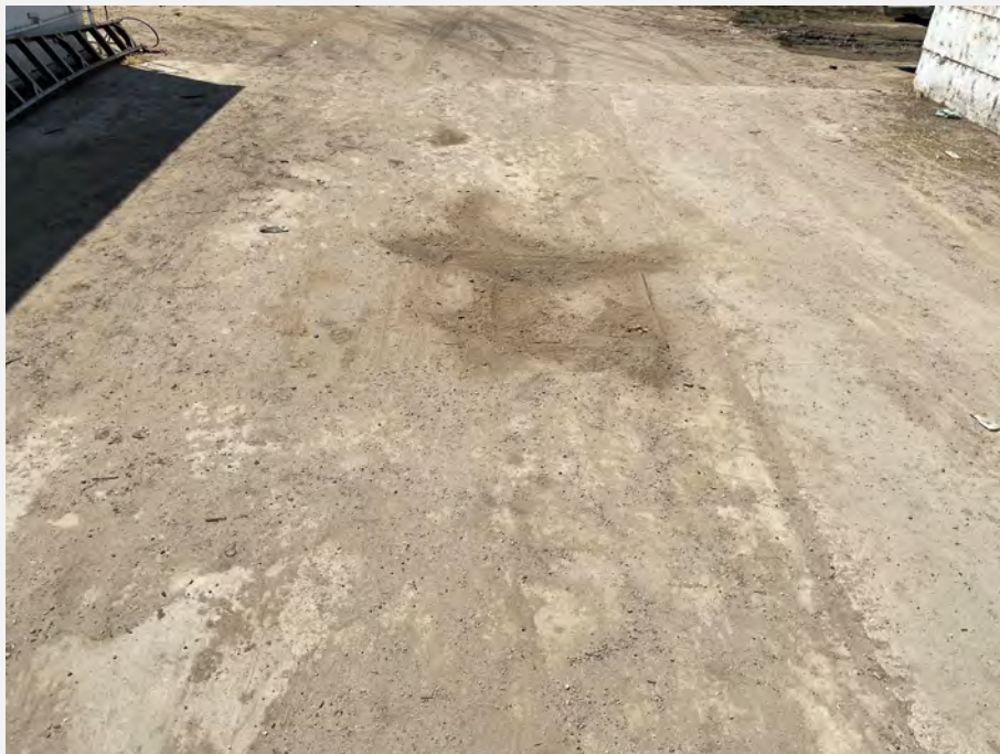
48. Floor drain filled in with soil located in concrete pad between the two outbuildings behind the residential structures at 12607 and 12609 Avenue 228.
