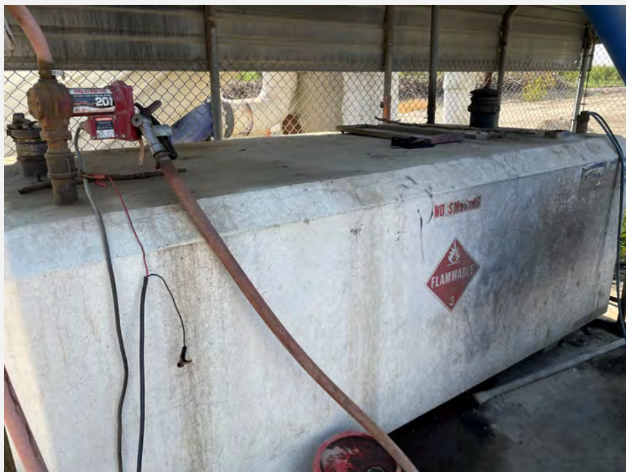
32. Diesel Fuel AST located adjacent to the irrigation supply groundwater well. Estimated to be approximately 1,000 gallons.
