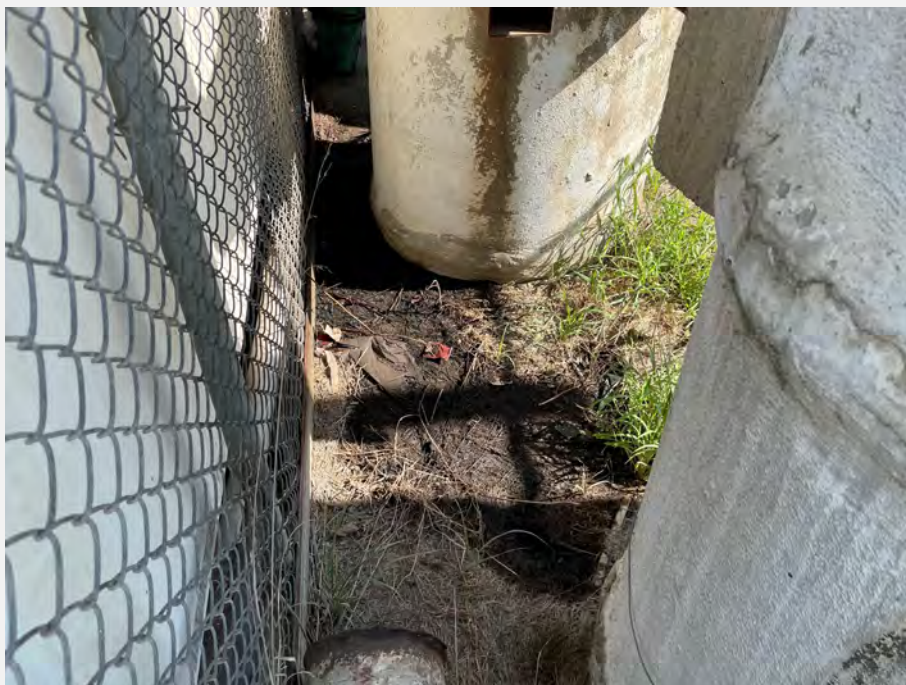
34. Soil staining observed adjacent to surface casing of irrigation supply groundwater well.
