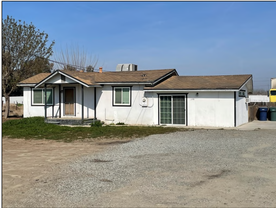
View of the single-family residence looking north across the site.
