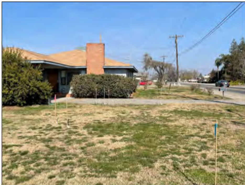
View of the ROW and TCE take areas looking north from the southwest corner of the property.
