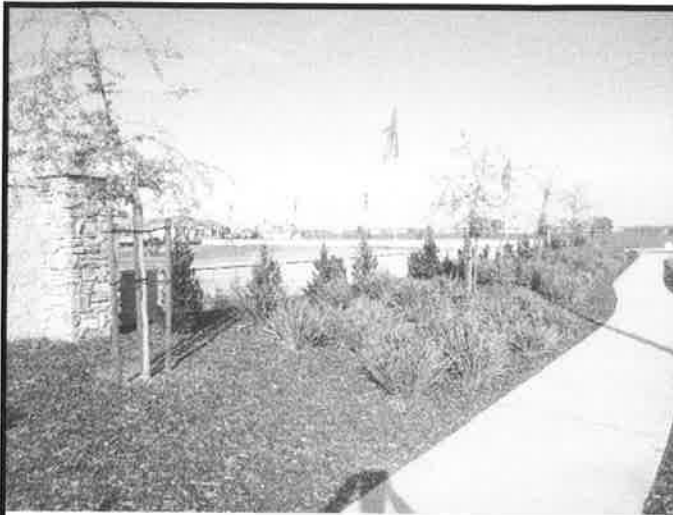
DEVONSHIRE STREET HALF HEIGHT BLOCK WALL
