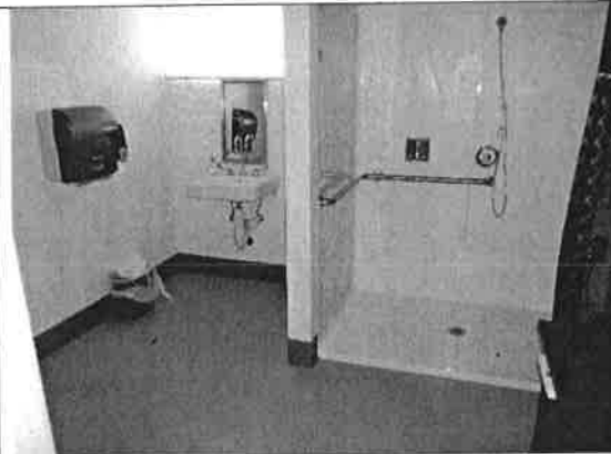
Bathroom with shower
